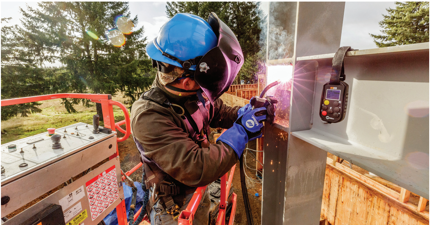
Fig. 1 — Wireless Interface Control for the Trailblazer® and Big Blue® places full control of the welding machine/generator in the palm of the operator's hand, so he or she can remotely adjust amperage and voltage, customize welding programs, turn the machine on and off, select processes, and fine-tune the welding arc.
